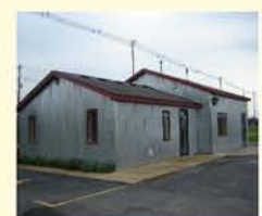
Rear of Building
